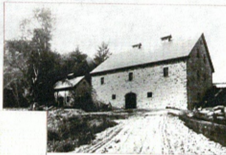
Wine cellar built by Gier in 1903 (now the Hess Collection Winery).
