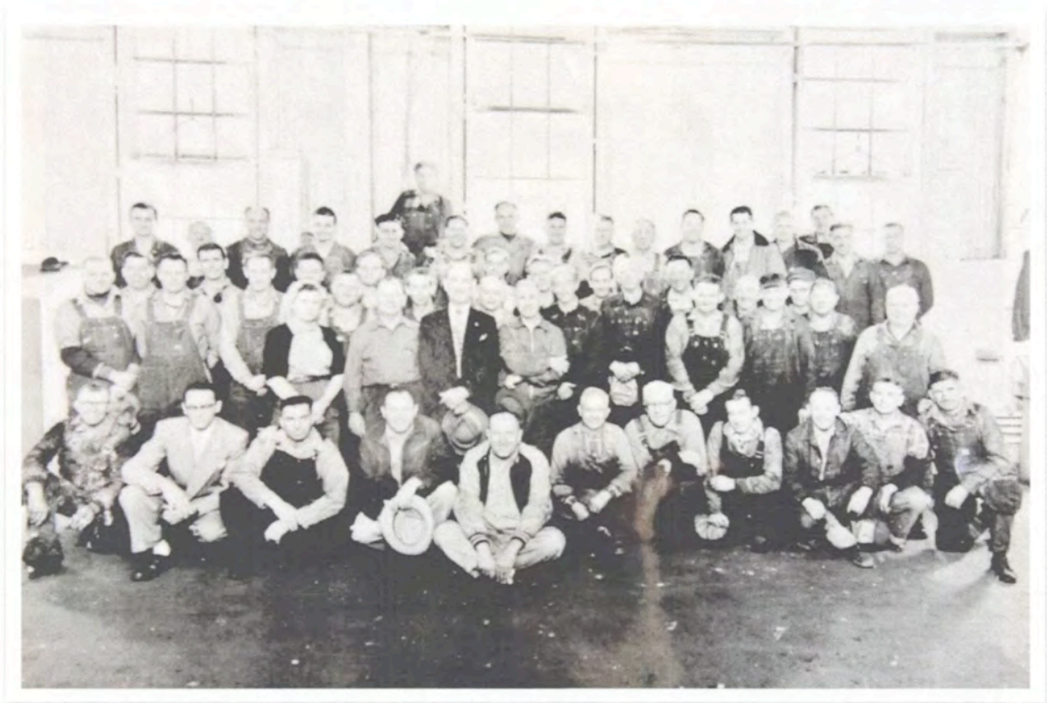
Southern Pacific Pipe Shop, Sacramento, CA 1946
