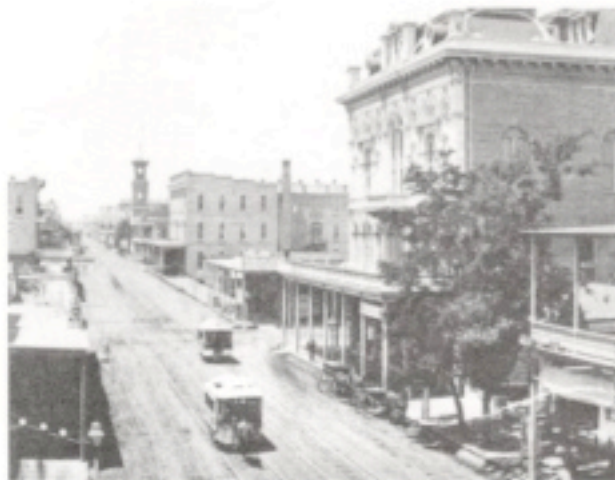
Mule-drawn streetcars at Eighth and K Streets on Sacramento's newly raised streets, circa 1870. Author's collection.
