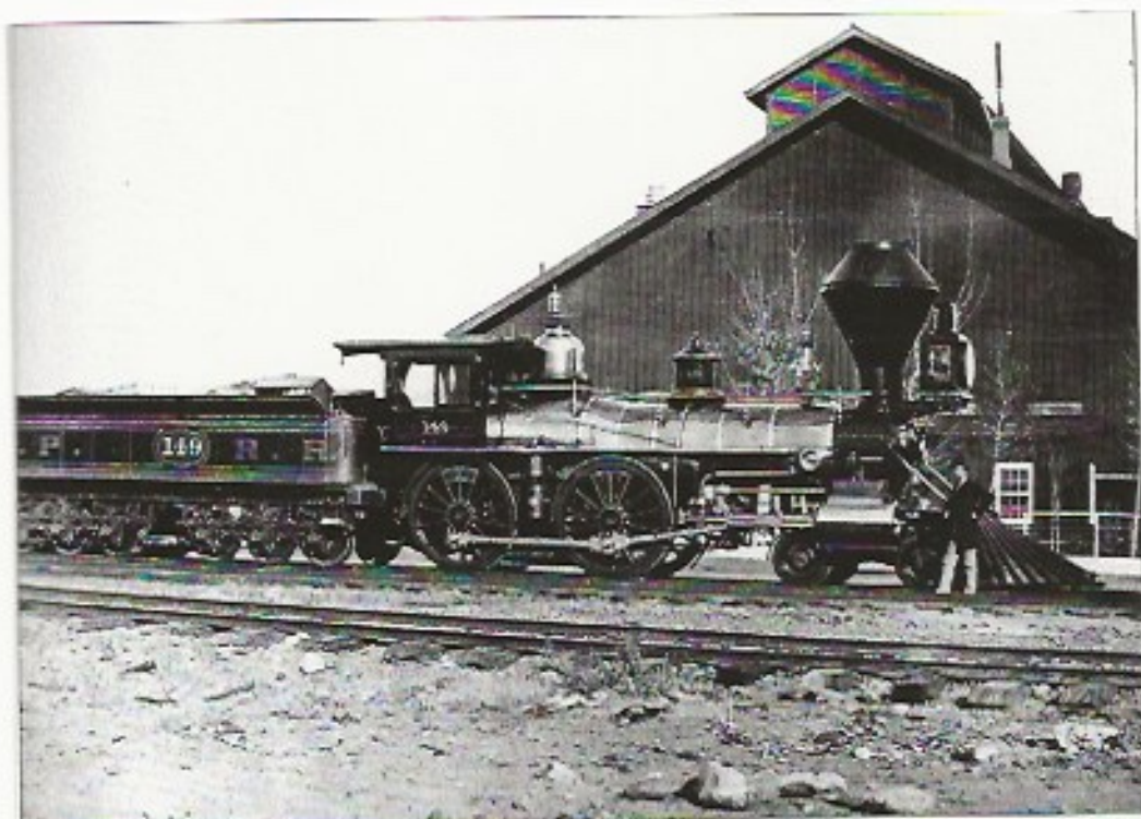
Central Pacific locomotive No. 149, sporting an enlarged tender fabricated at the Sacramento shops, stands in Wadsworth, Nevada, in the 1870s. The tender's larger fuel and water capacity helped No. 149 cover the Ogden, Utah-to-Oakland leg of Jarrett and Palmer's Lightning Express , which brought the theatrical production of "Henry V" from New York to San Francisco in a mere 84 hours. (Courtesy of the California History Room, California State Library, Sacramento.)
