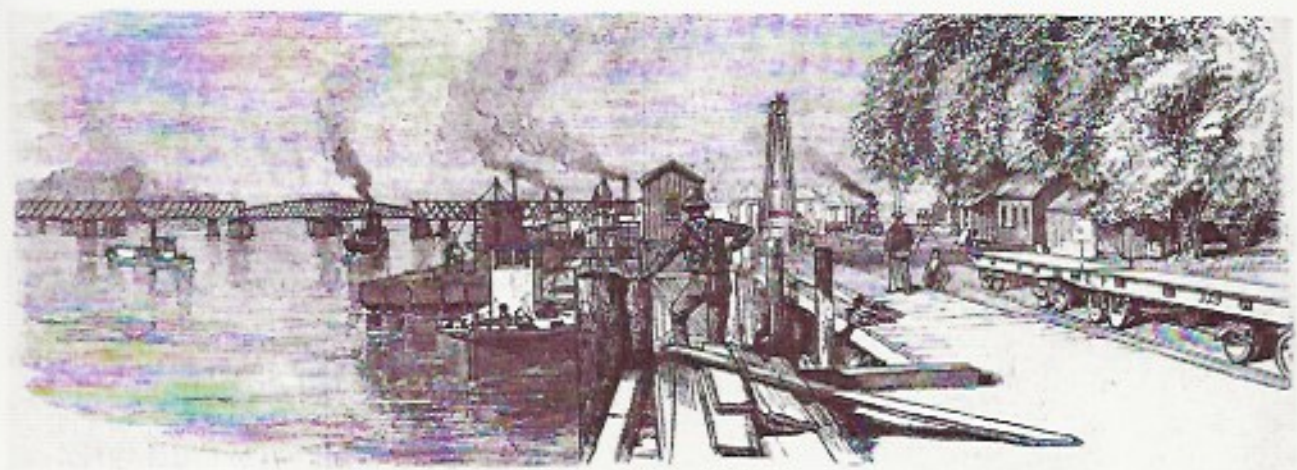
The new railroad bridge across the Sacramento River formed a background for dockside activity SCCL
