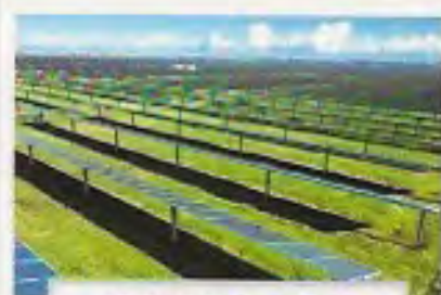
30 Meg Solar Power Plant
