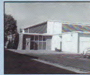
SEPTEMBER 1956 → School opened with administration and classroom wings completed. Three months later the gymnasium, science laboratories and cafeteria were completed.
