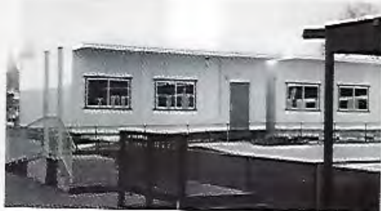
The portables are getting ready to be moved.
