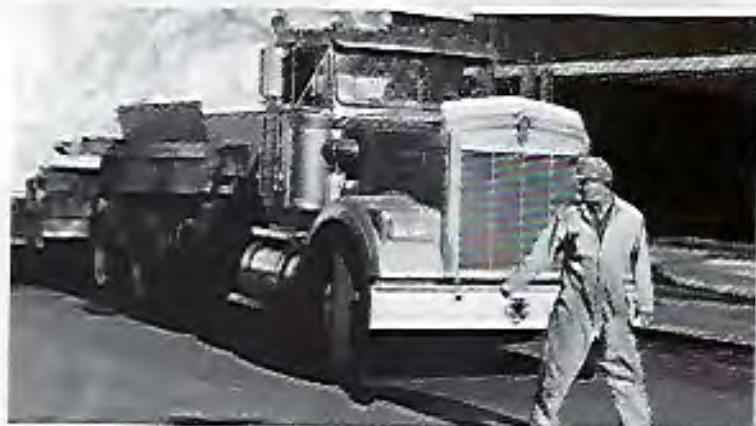
Construction worker shown guiding the mover.
