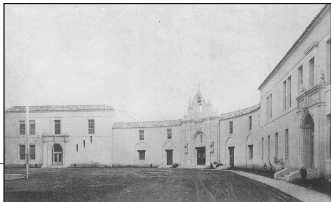
The just completed school at 21st Street, 1925
