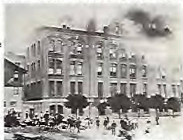
Saint Mary's College suffered a second fire in 1918.
